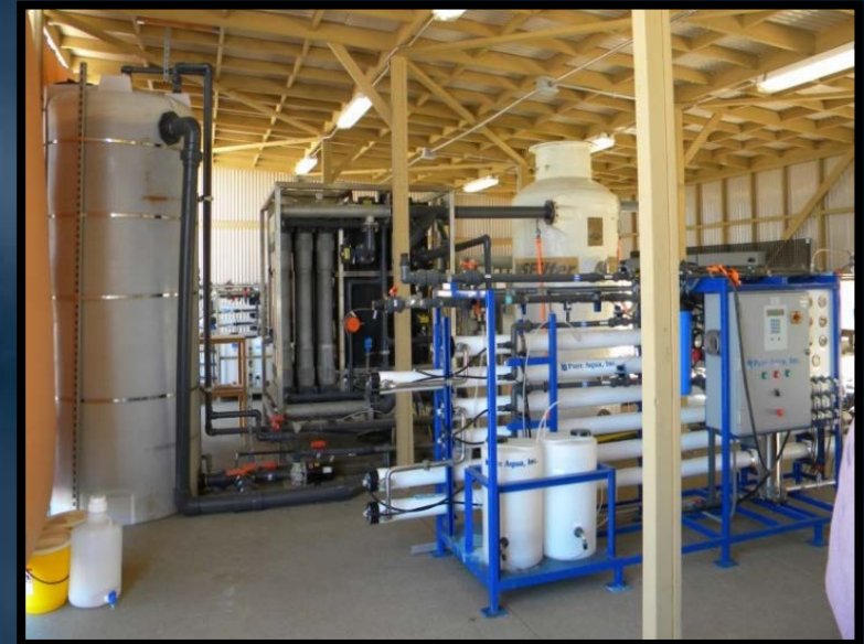
Pilot Plant at JWPCP
